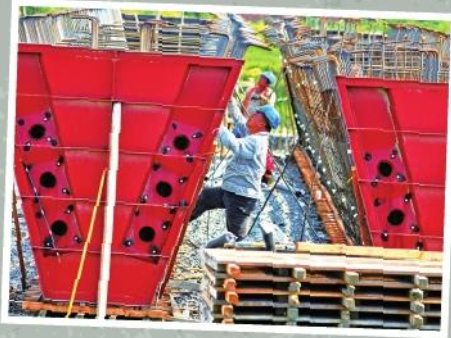
④ build bridges
