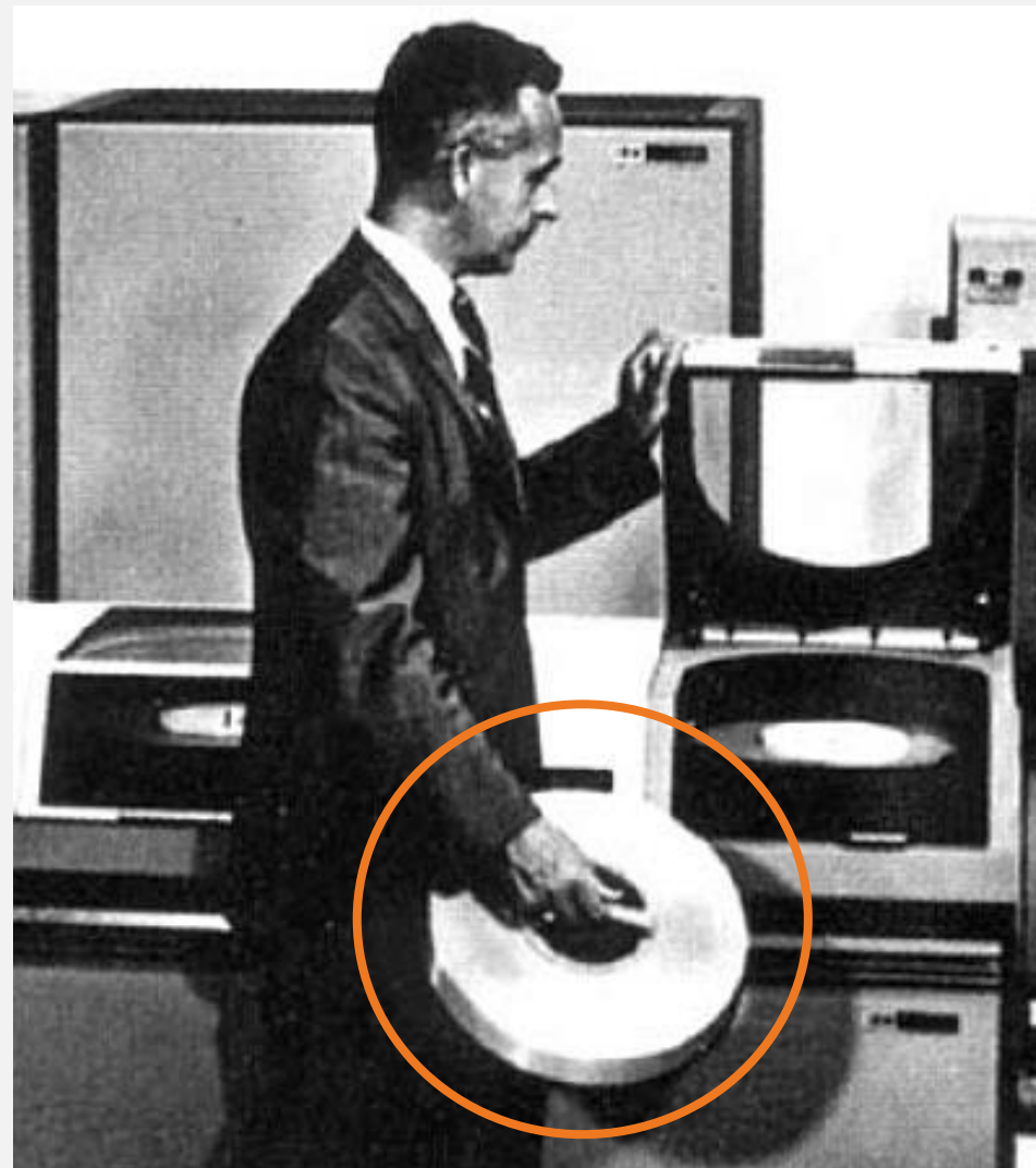
1974, IBM 3340 ( Winchester) 35 or 70Mb , 14-inch
